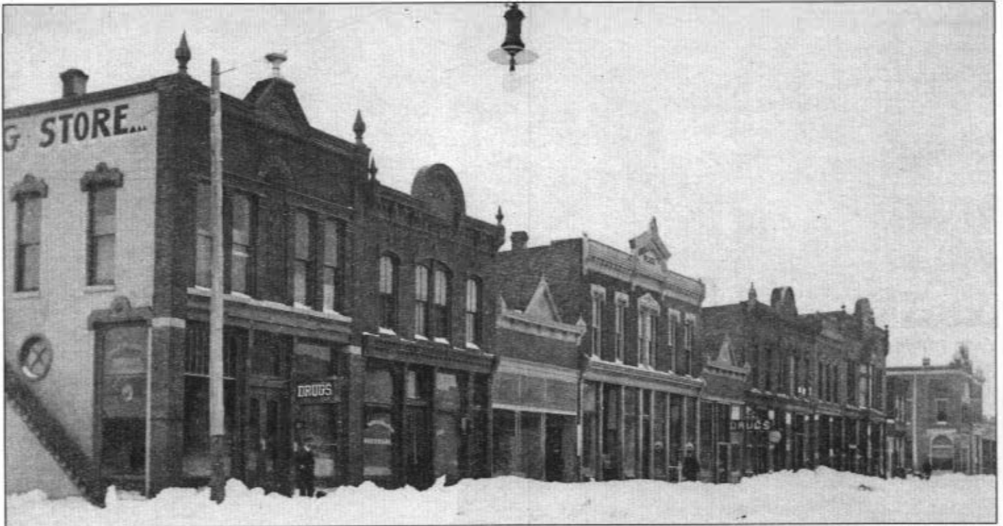
This photograph is of the south side of the St. Paul business district in February of 1915. Polansky's Drug Store is at the east end of the block (left) with Johnson & Sons Hardware next to it. Another drug store is located in the middle of the block.
