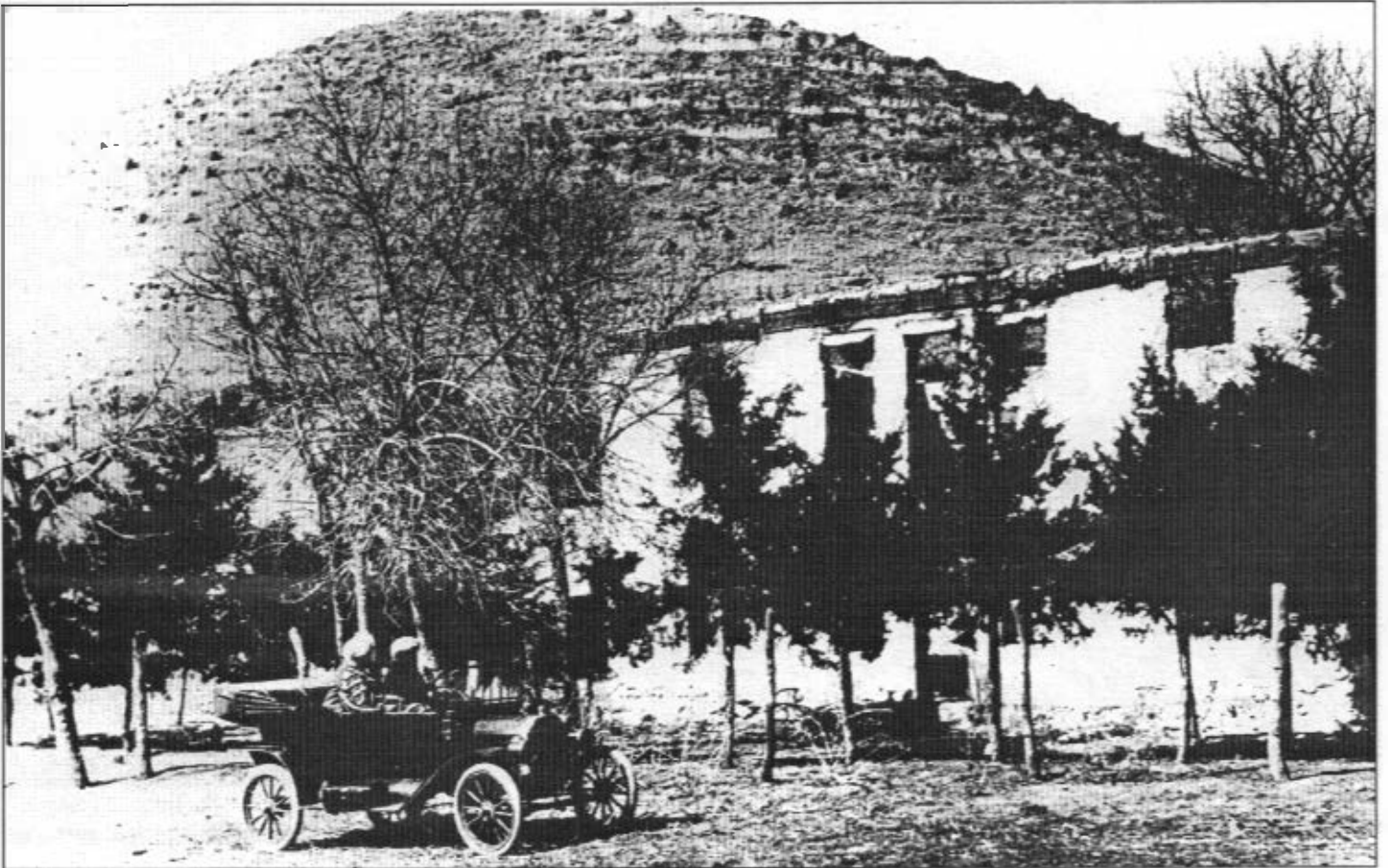
Joseph "Doc" Beebe constructed a hotel using a quick-lime product from his kilns east of Cotesfield. He used the same technique used to build the buildings at Fort Hartsuff. His hotel was known as the "Concrete Hotel" or the "Half-Way House" and was located east of Cotesfield, one mile south of the present river bridge. The couple is believed to be the Leschinskys, who had a photography studio in Grand Island.
