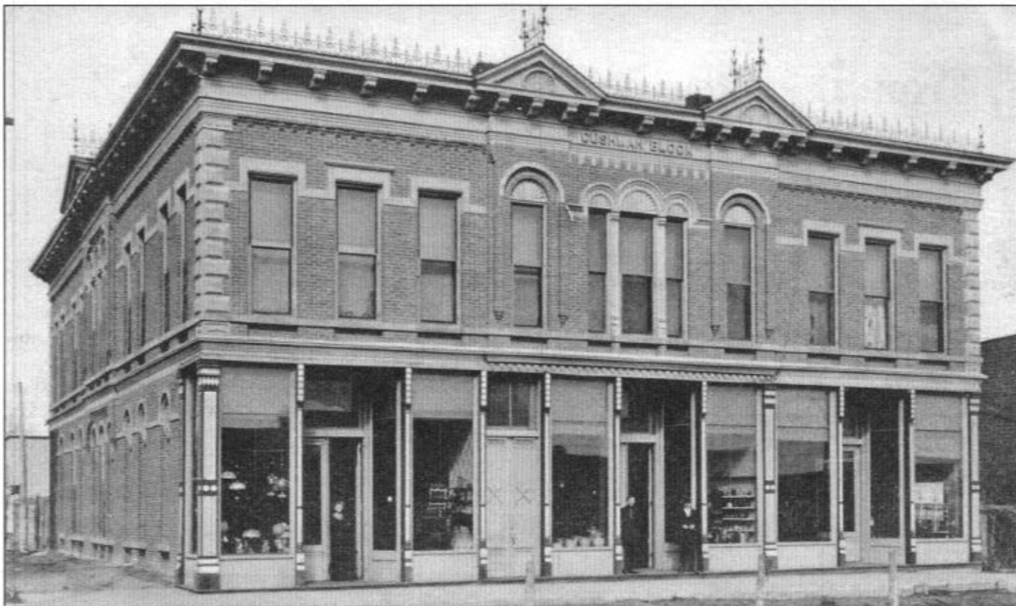
A number of businesses appear to be located on the first floor of the Cushman building at 6th and Howard. This building was originally a hotel.
